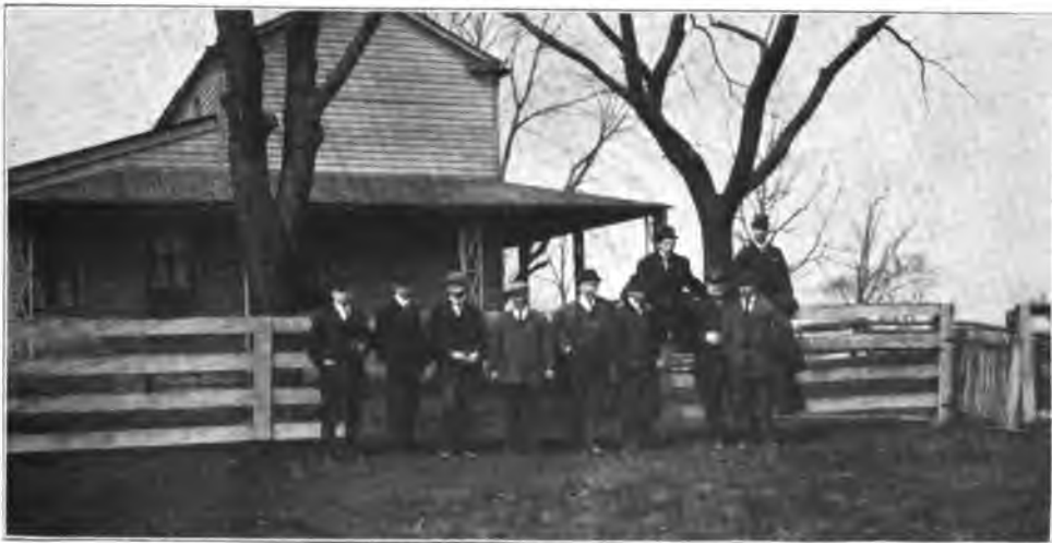
TEMPORARY LOCKER HOUSE AT BEVERLY
